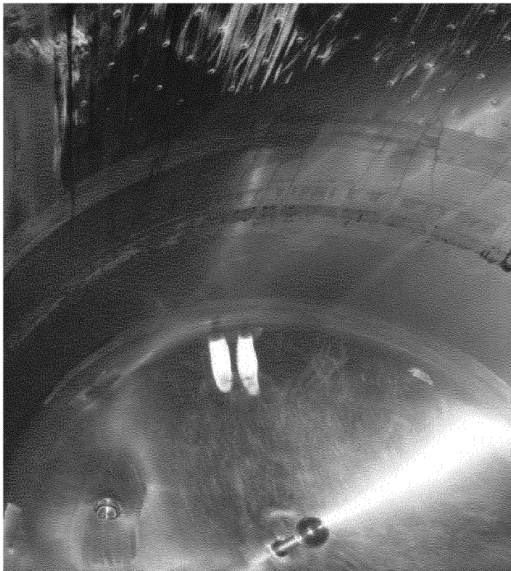
Tank before cleaning
