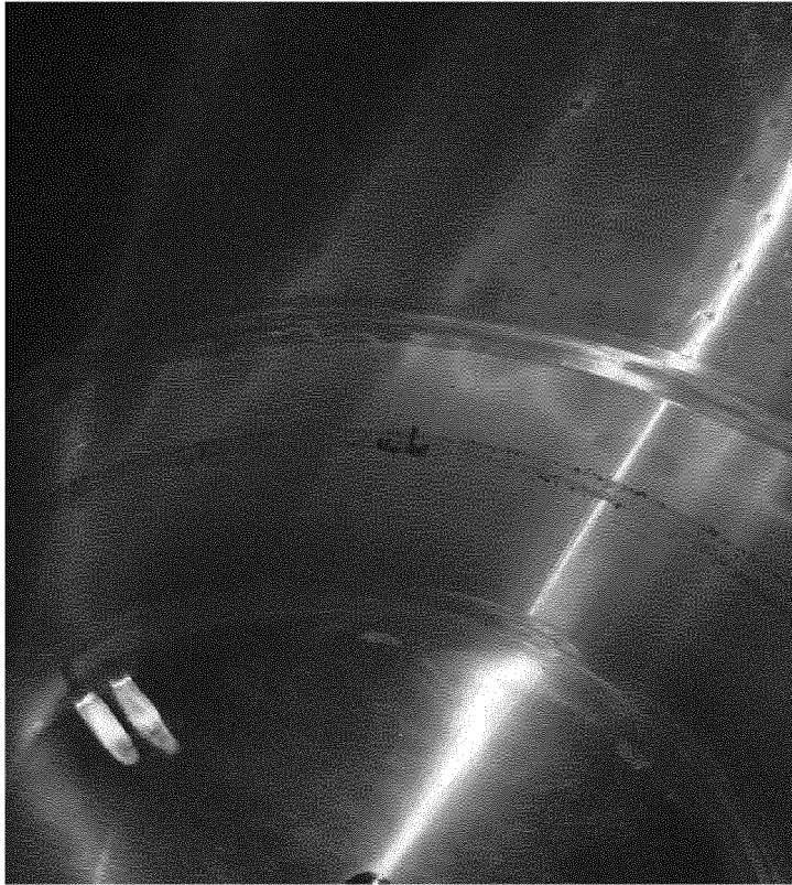
Tank after cleaning
