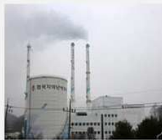
Combined heat and power (CHP) plant
